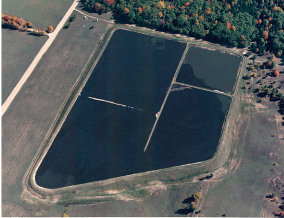
Figure 21. Dredged sediment disposal cell (aerial view).
