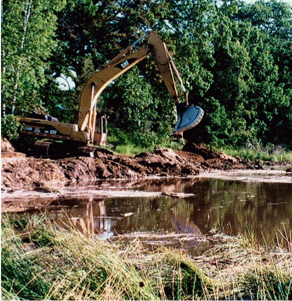
Figure 19. Dredging with a backhoe.
